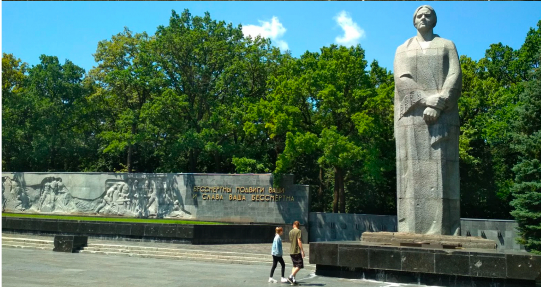
Damaged wall in Kharkiv Glory Memorial Site
