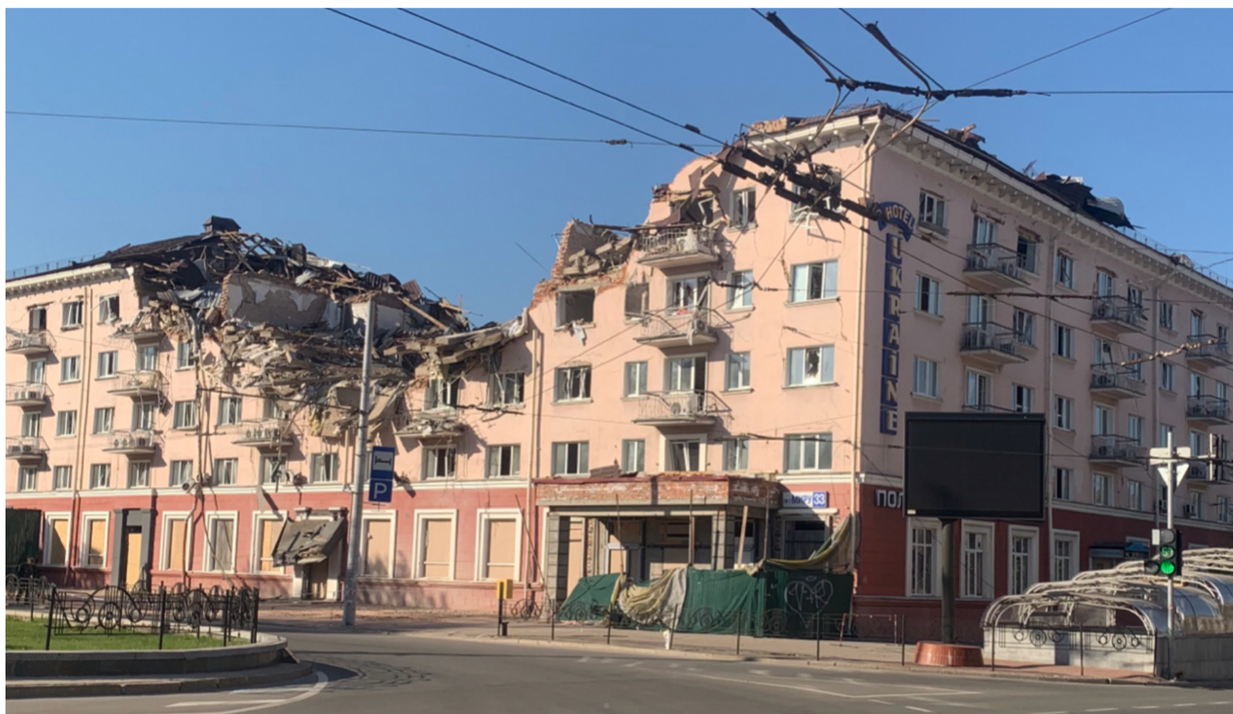
Chernihiv, an apartment house in the city center.
